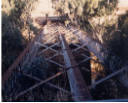
B7055 Glenmona Bridge
