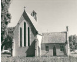
B3355 St Paul's Church Front View
