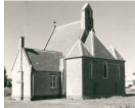
B3355 St Paul's Church Back View
