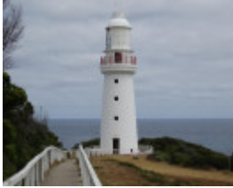
B2320 Cape Otway Lighthouse
