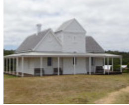
B2320 Cape Otway telegraph station
