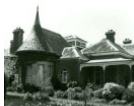
B1709 Coragulac House South Side
