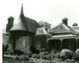
B1709 Coragulac House South Side
