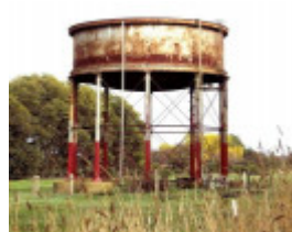
B4458 Railway Station Watertower
