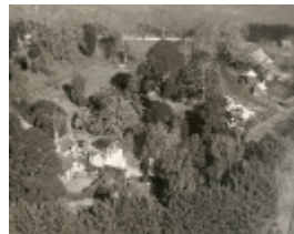
B1066 Ripple Vale Homestead & Outbuildings
