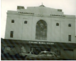
B5116 RSL Building
