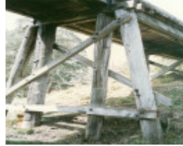
B3711 Curdies River Railway Bridge
