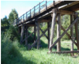
B3711 Curdies River Railway Bridge
