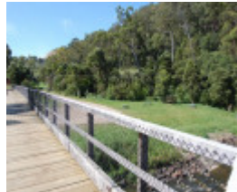
B3711 Curdies River Railway Bridge Deck
