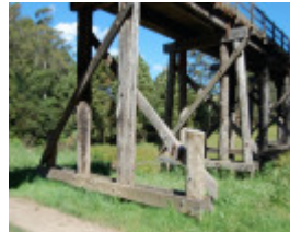
B3711 Curdies River Railway Bridge
