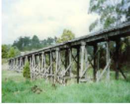
B3711 Curdies River Railway Bridge
