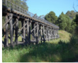
B3711 Curdies River Railway Bridge
