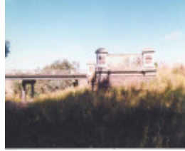
B7003 Old Darlington Bridge & Abutments
