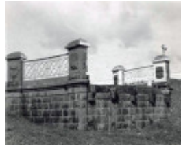
B7003 Old Darlington Bridge & Abutments
