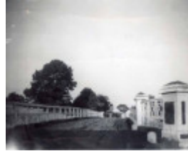
B7003 Old Darlington Bridge & Abutments
