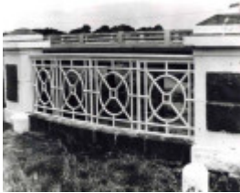
B7003 Old Darlington Bridge & Abutments
