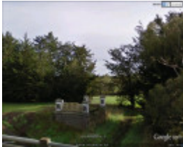
B7003 Old Darlington Bridge & Abutments
