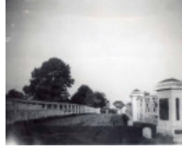
B7003 Old Darlington Bridge & Abutments
