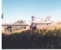
B7003 Old Darlington Bridge & Abutments
