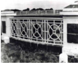
B7003 Old Darlington Bridge & Abutments
