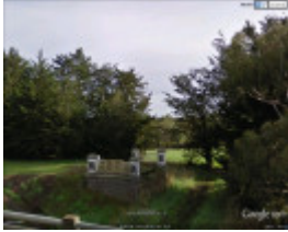
B7003 Old Darlington Bridge & Abutments
