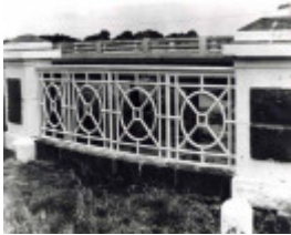
B7003 Old Darlington Bridge & Abutments
