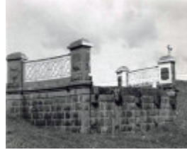
B7003 Old Darlington Bridge & Abutments
