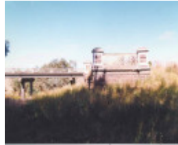
B7003 Old Darlington Bridge & Abutments
