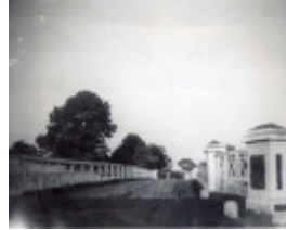
B7003 Old Darlington Bridge & Abutments
