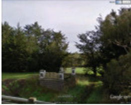
B7003 Old Darlington Bridge & Abutments
