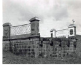
B7003 Old Darlington Bridge & Abutments
