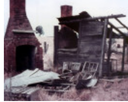
B2938 Kelly House Chimney
