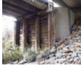
B 6845 Bete Bolong abutment
