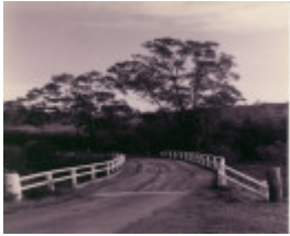
B6845 Bete Bolong Creek Bridge
