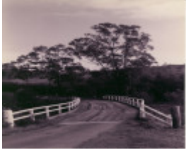
B6845 Bete Bolong Creek Bridge
