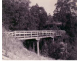
B6845 Bete Bolong Creek Bridge
