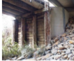
B 6845 Bete Bolong abutment
