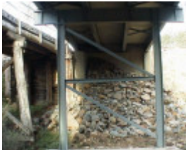
B6845 Bete Bolong substructure
