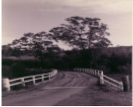
B6845 Bete Bolong Creek Bridge
