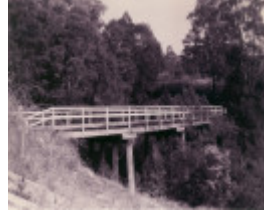
B6845 Bete Bolong Creek Bridge
