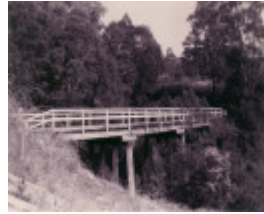
B6845 Bete Bolong Creek Bridge
