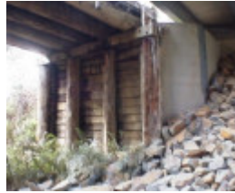
B 6845 Bete Bolong abutment
