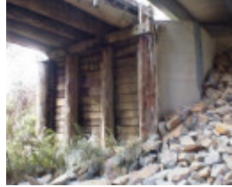
B 6845 Bete Bolong abutment
