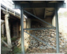
B6845 Bete Bolong substructure
