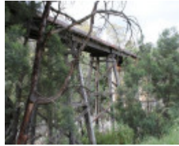
B6943 Boggy Creek Bridge Piers
