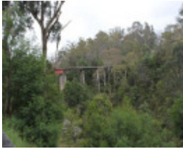
B6943 Boggy Creek Bridge
