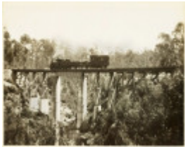
B6943 Boggy Creek Bridge 1915
