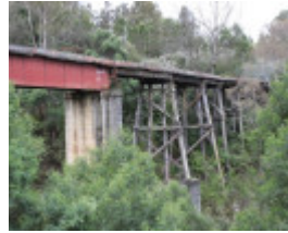
B6943 Boggy Creek Bridge
