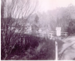
B7056 Cobungra River Bridge
