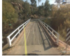
B7056 Cobungra River Bridge (Google Earth Image)
