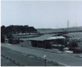
B6788 Former Railway Goods Shed
