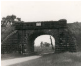
B2551 Bluestone Bridge
