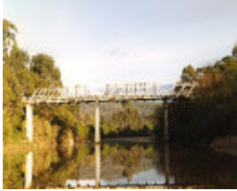
B2260 Genoa River Bridge
