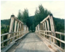
B2260 Genoa River Bridge
