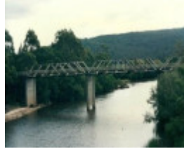
B2260 Genoa River Bridge
