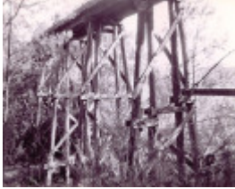
B6947 Hospital Creek No1 Bridge
