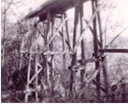
B6947 Hospital Creek No1 Bridge
