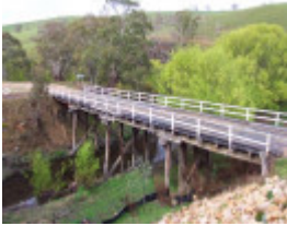
B6842 Jubilee Bridge
