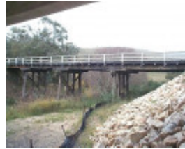
B6842 Jubilee Bridge side
