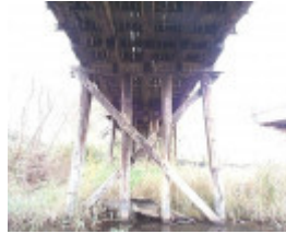
B6842 Jubilee Bridge Omeo piers
