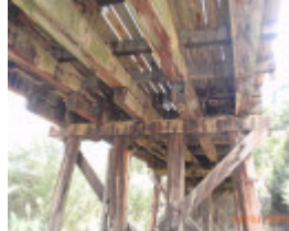
B6842 Jubilee Bridge substructure
