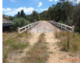
B6842 Jubilee Bridge deck
