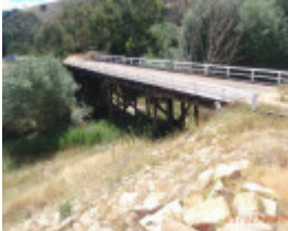
B6842 Jubilee Bridge
