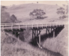
B6842 Jubilee Bridge
