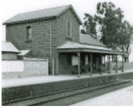
B2354 Railway station Lethbridge
