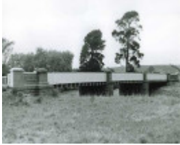
B3263 Iron Bridge
