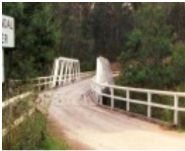
B6847 Murrindal Bridge
