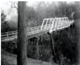
B6847 Murrindal Bridge
