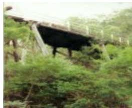
B6847 Murrindal Bridge
