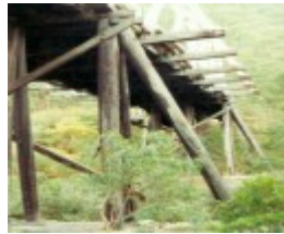
B6847 Murrindal Bridge
