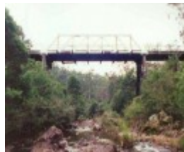
B6847 Murrindal Bridge
