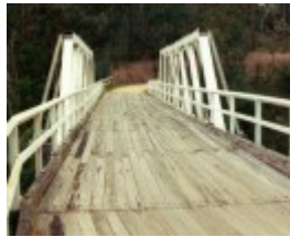
B6847 Murrindal Bridge
