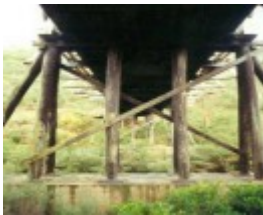
B6847 Murrindal Bridge
