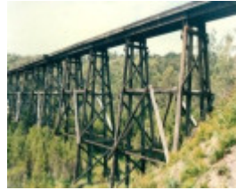
B3484 Stony Creek Bridge
