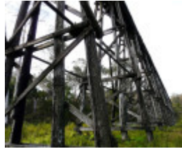
B3484 Stony Creek Bridge
