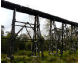
B3484 Stony Creek Bridge
