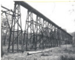
B3484 Stony Creek Bridge
