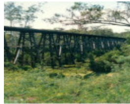
B3484 Stony Creek Bridge
