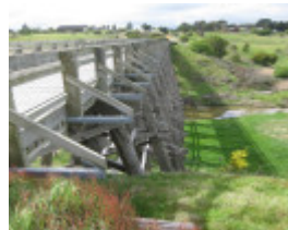
B7086 Nimons Bridge deck 2011
