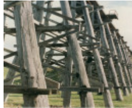
B7086 Nimons Bridge piers
