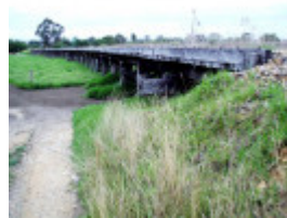
B6948 Snowy River Floodplain Bridges
