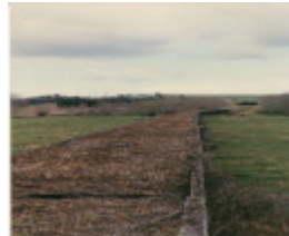
B6948 Short Bridge 1994
