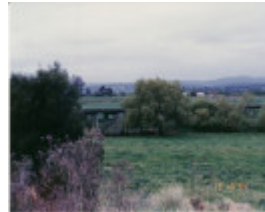
B6948 Long Bridge West End
