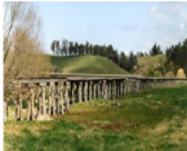
B6948 Longer of the Snowy River Floodplain Railway Bridges
