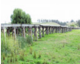
B6948 Snowy River Floodplain Bridges
