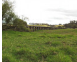
B6948 Snowy River Floodplain Bridges
