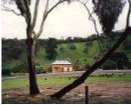
B0779 Shop & Residence Steiglitz
