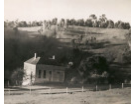
B0779 Shop & Residence Steiglitz
