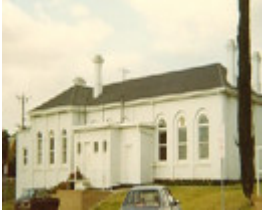
B5526 Water Tank & Plant
