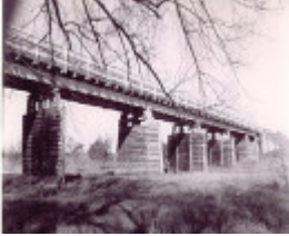
B6908 Wuk Wuk Bridge
