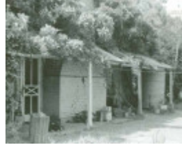
B1090 Gonn Crossing Homestead Rear View
