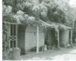
B1090 Gonn Crossing Homestead Rear View
