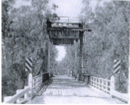
B7214 Gonn Crossing Bridge
