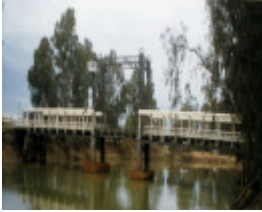
B4916 Barham-Koondrook Lift Bridge
