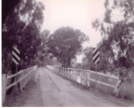
B6925 Tragedy Bridge 1996
