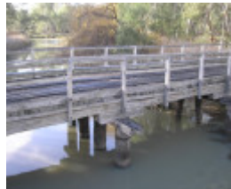
B6925 Tragedy Bridge side view
