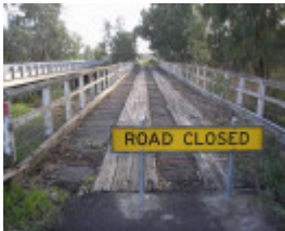
B6925 Tragedy Bridge 2009
