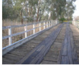
B6925 Tragedy Bridge deck
