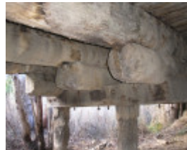
B6925 Tragedy Bridge substructure
