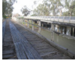
B6925 Tragedy Bridge
