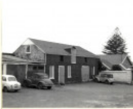
B0865 House Portland
