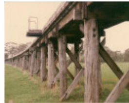
B6940 Wannon River Bridge
