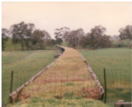
B6940 Wannon River Bridge
