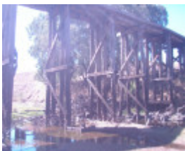
B6940 Wannon River Bridge
