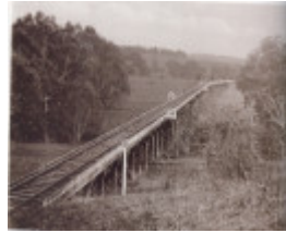
B6940 Wannon River Bridge
