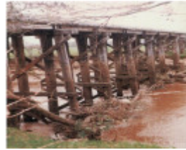
B6940 Wannon River Bridge
