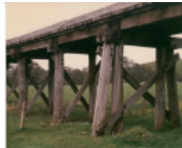
B6940 Wannon River Bridge
