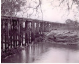
B6940 Wannon River Bridge
