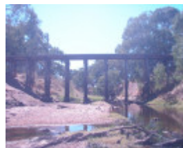
B6940 Wannon River Bridge Casterton
