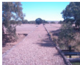
B6940 Wannon River Bridge Casterton
