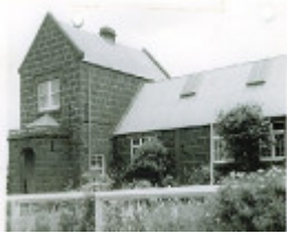
B0053 Former National School Portland
