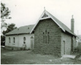
B0055 St Stephen s Anglican Parish Hall Portland
