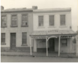
B0882 114 116 Percy St Portland 116 Demolished
