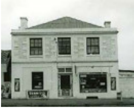
B0891 Federal House Portland
