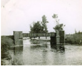
B2212 Hotspur Bridge
