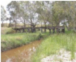
B6944 Dwyer's Creek Bridge
