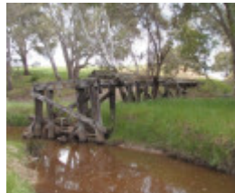
B6944 Dwyer's Creek Bridge
