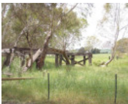
B6944 Dwyer's Creek Bridge
