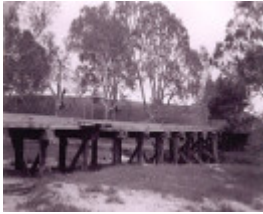
B6944 Dwyer's Creek Bridge
