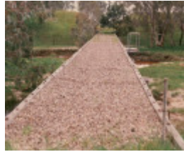
B6944 Dwyer's Creek Bridge
