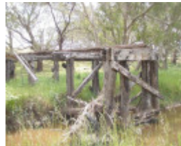
B6944 Dwyer's Creek Bridge
