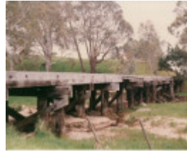
B6944 Dwyer's Creek Bridge
