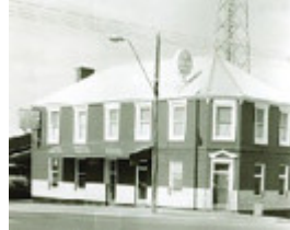
B0879 Royal Hotel after verandah removed
