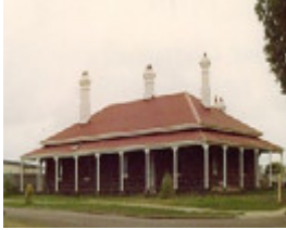
B2323 Lighthouse Keeper's Cottage Portland
