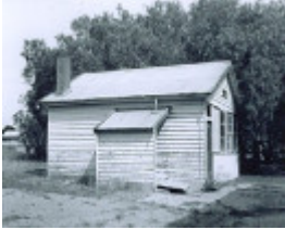
B4639 Portable Rural School Building
