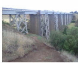
B5142 Moorabool viaduct
