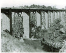
B5142 Moorabool Viaduct
