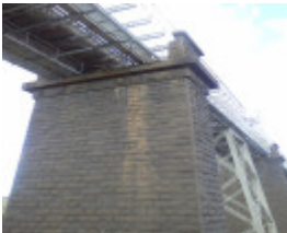
B5142 Moorabool viaduct
