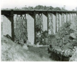
B5142 Moorabool Viaduct
