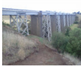
B5142 Moorabool viaduct
