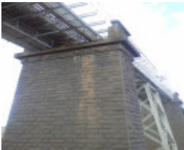
B5142 Moorabool viaduct
