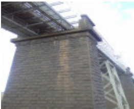
B5142 Moorabool viaduct
