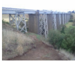
B5142 Moorabool viaduct
