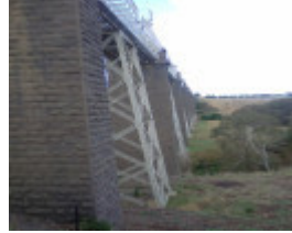
B5142 Moorabool viaduct
