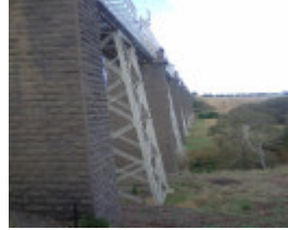
B5142 Moorabool viaduct
