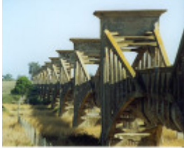
B5779 Ovoid Sewer Aqueduct
