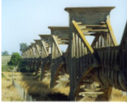
B5779 Ovoid Sewer Aqueduct
