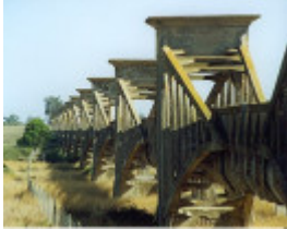
B5779 Ovoid Sewer Aqueduct
