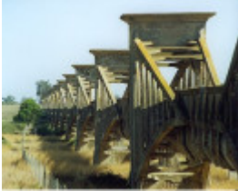
B5779 Ovoid Sewer Aqueduct
