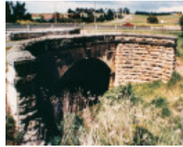
B2643 Waurn Ponds Bridge
