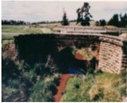
B2643 Waurn Ponds Bridge
