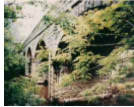
B1339 Bluestone Bridge Ballarat Rd Batesford
