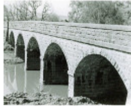
B1339 Bluestone Bridge
