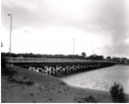
B6798 Barwon Heads Bridge
