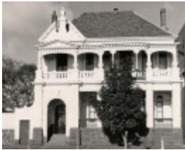
B3771 Fmr Corio Terrace
