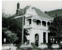
B3771 Fmr Corio Terrace
