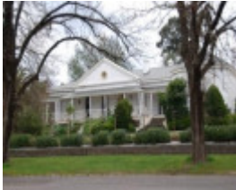
B0047 Bungalow - Former Post Office
