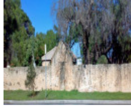
B5045 Former Lake Bank Hotel Showing former Shelter for Itinerate Travellers
